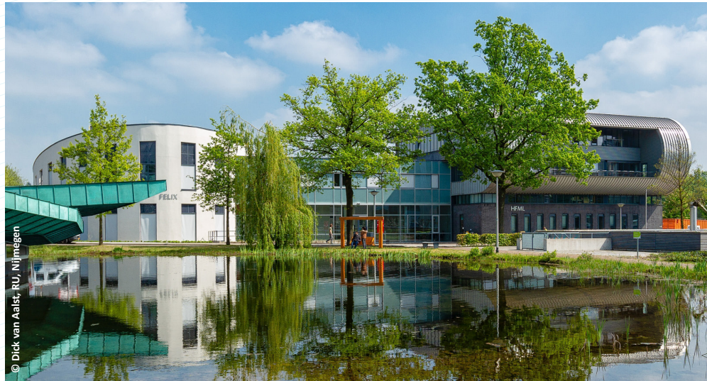
The combined HFML-FELIX building.
