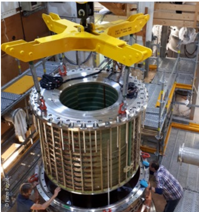
› Figure 1: Successful insertion of the superconducting coil in the He vessel. In the most constraint part, the radial clearance is 0.4 mm.
