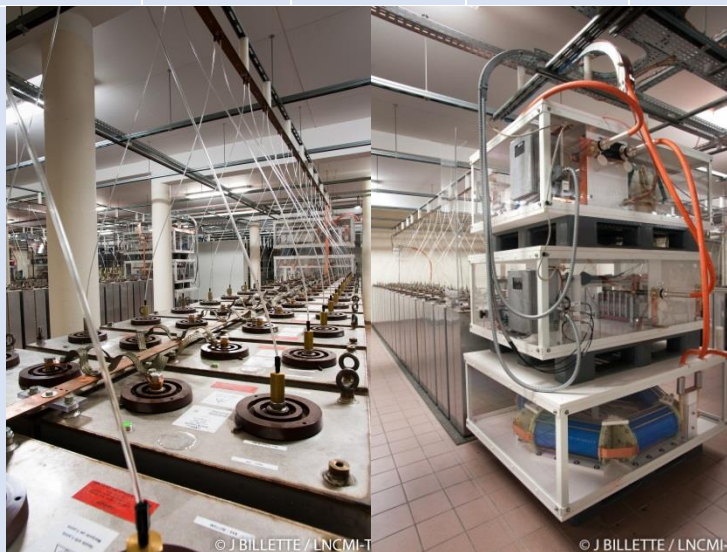
Pictures of one 3.5 MJ module of the 14 MJ generator
